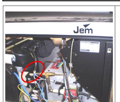
3. Before fitting the Fuse Plate assembly, you will first need to disconnect and remove the live (brown) heater wire from the upper spade of the relay that goes to the PCB. Remove the cable ties so that the wire can be fed through and disconnect from the 'piggy-back' crimp on the relay end.
