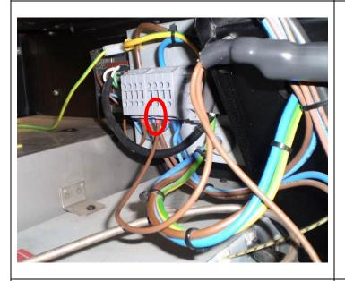
10. Connect the red pin on the end of the Brown wire to the remaining hole on the distribution block as shown.
