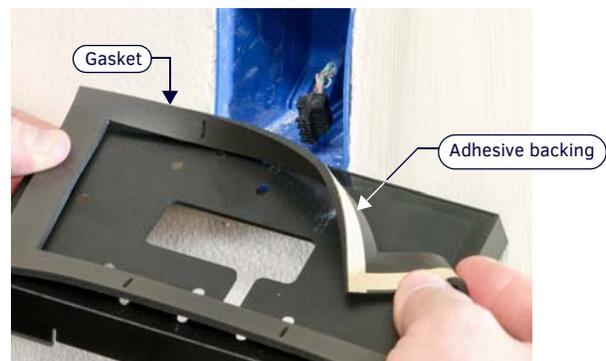
FIG. 4 APPLYING THE OPTIONAL FOAM GASKET TO THE BACK BOX.
