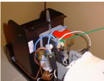
Thermal wire & the blue wire from the pcb in place on the heater leg.
